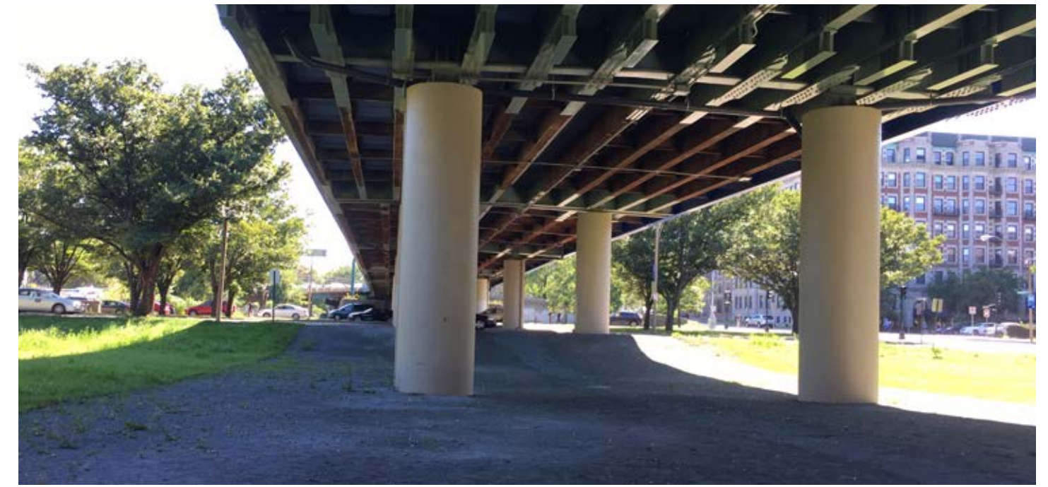
Photo of the existing condition of the North Field looking south.
