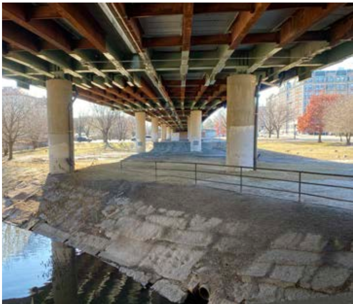
Removed viaduct wall.
