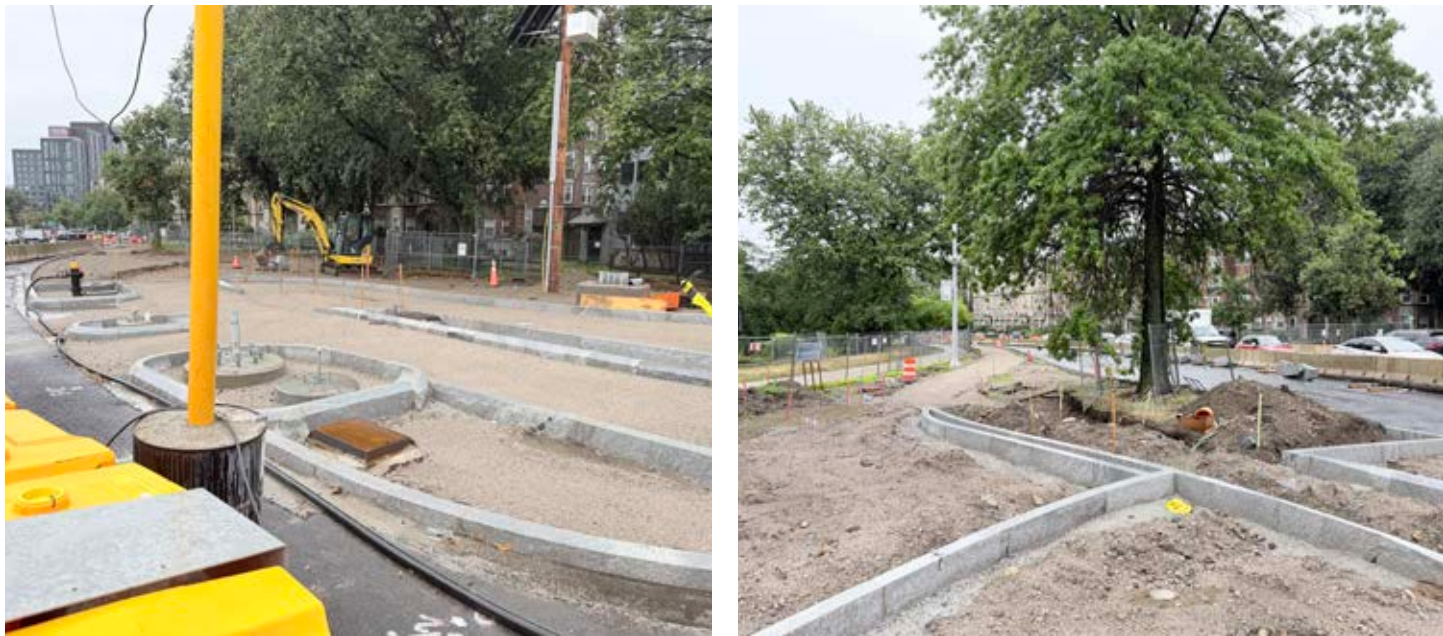
The new granite curbs are beginning to reveal the future layout of Charlesgate—expanding the park, narrowing the intersection, and creating dedicated walking and biking paths carefully laid out to preserve mature trees.
