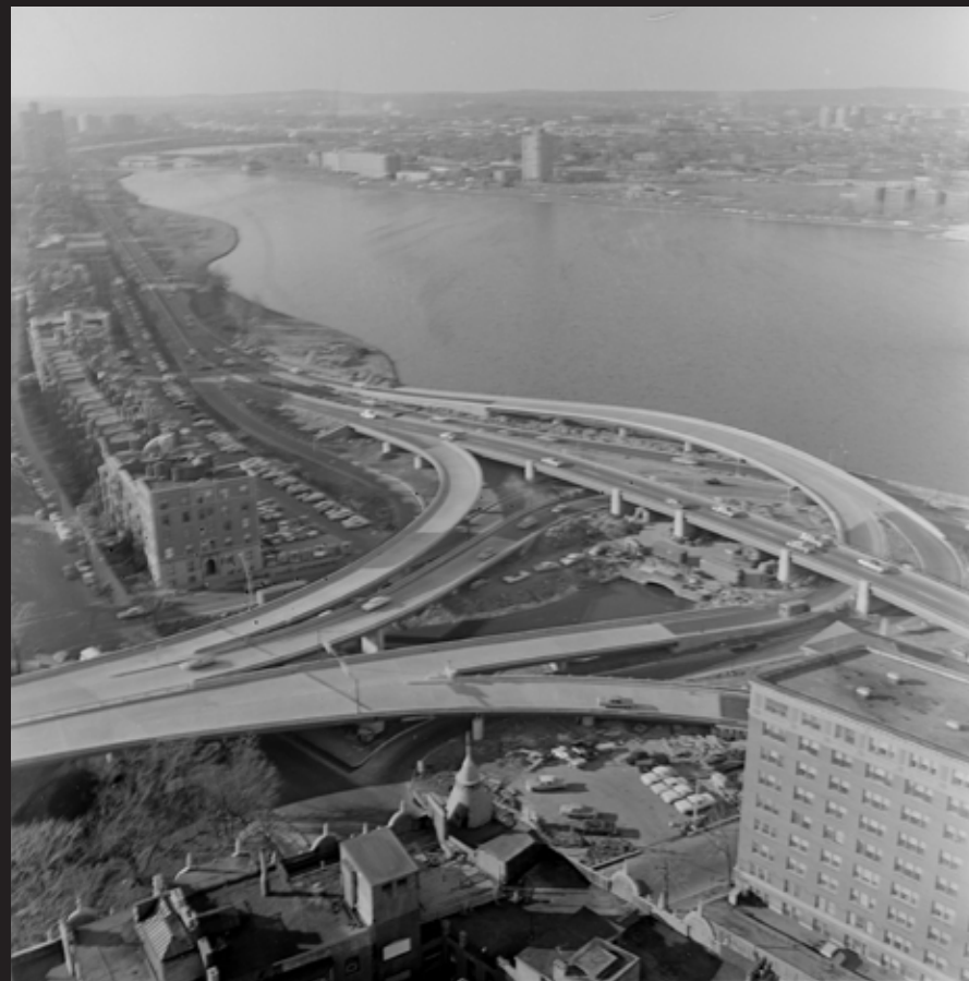
1966 photo of the Bowker and Storrow Dr. Bridges under construction. Digital Commonwealth.
