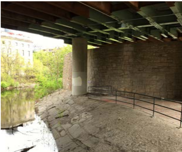
Existing viaduct wall.
