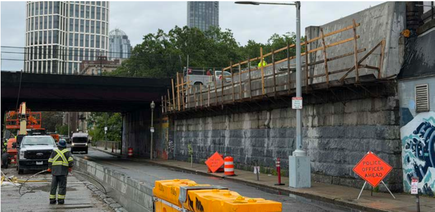
The new dedicated shared-use bridge and Charlesgate West bridge are being built directly on top of the original stone abutments from H.H. Richardson and Frederick Law Olmsted’s historic bridge.
