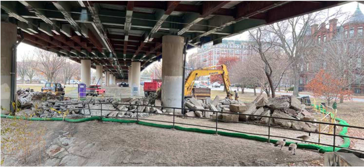
Wall removal in progress in the North Field.
