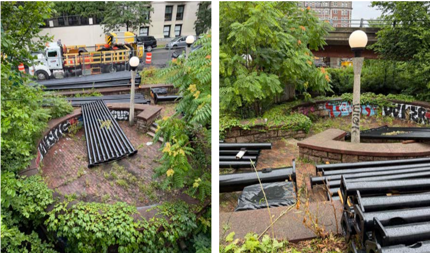
New light poles are being staged for installation along the new pedestrian pathways connecting the Back Bay Fens and Charlesgate Park.
