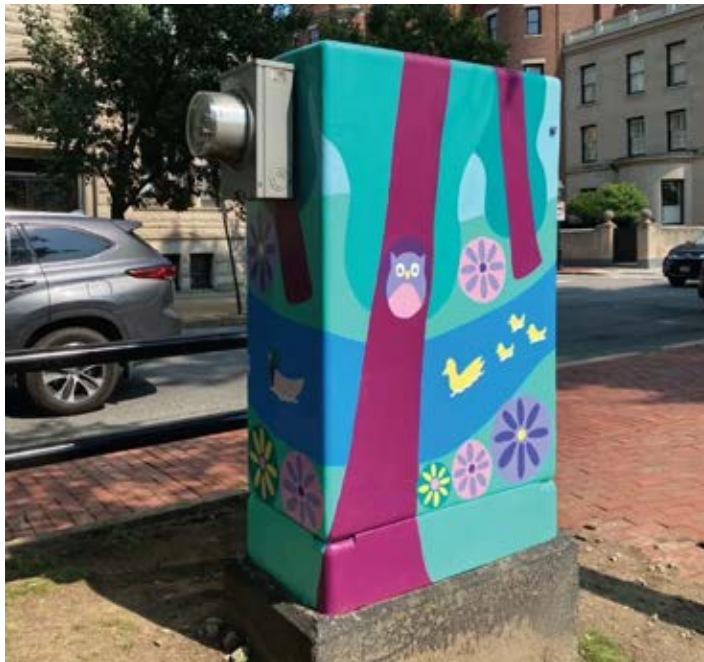
Finished utility box in the Grove.
