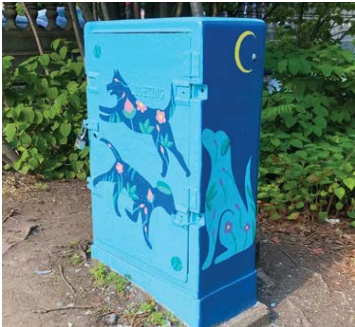
Finished utility box in the South Field.
